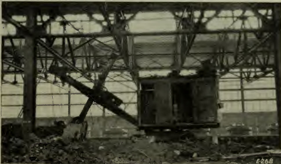
FIG. 12. GRADING WITH STEAM SHOVEL.
